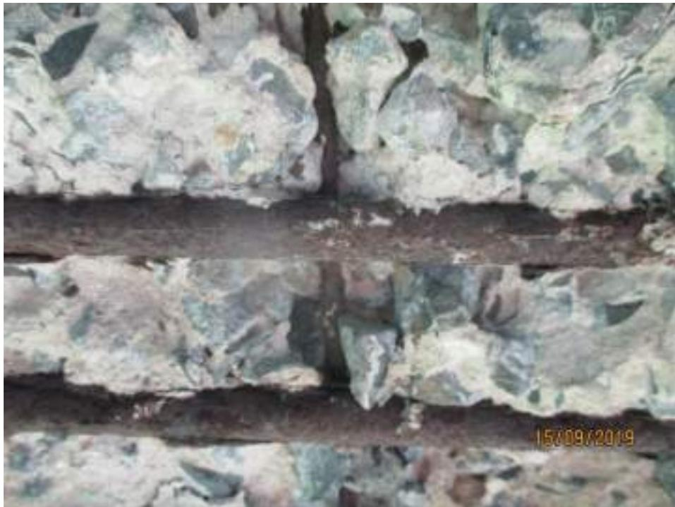
**Fig. 38 Visible of main reinforcement in RC element**
