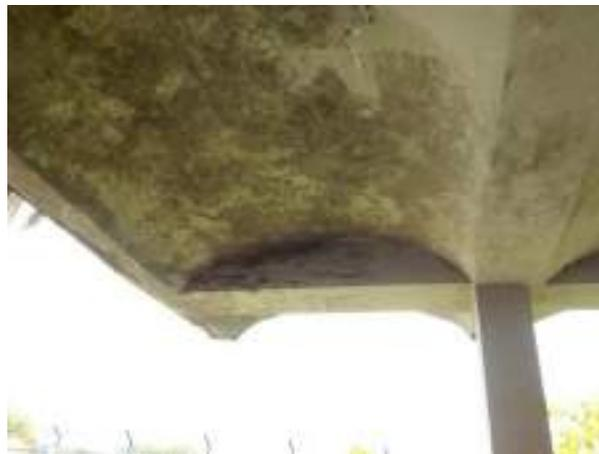
**Fig. 33: Cracks, spalling of concrete and dampness in the portico of CISF building**
