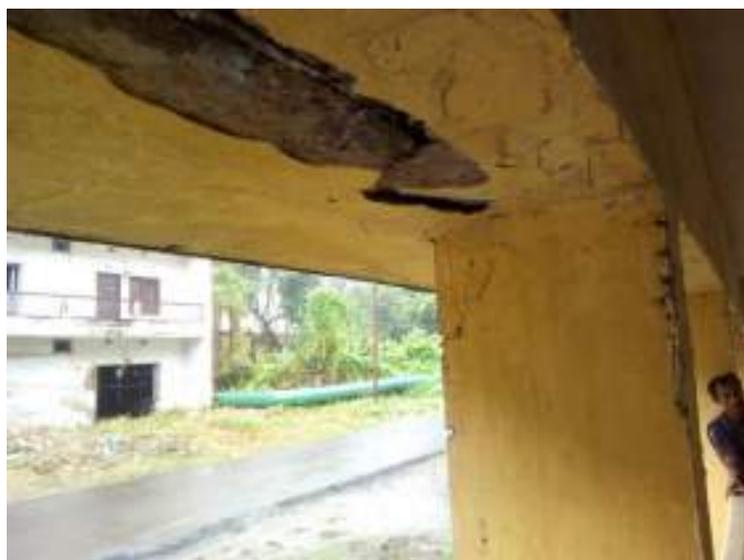
**Fig. 8: Crushing of Concrete in Ground Storey Column of Officers Hostel 1**
