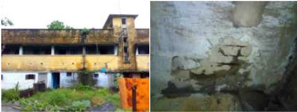
**Fig. 17: F Type Quarters (seepage from the roof)**
