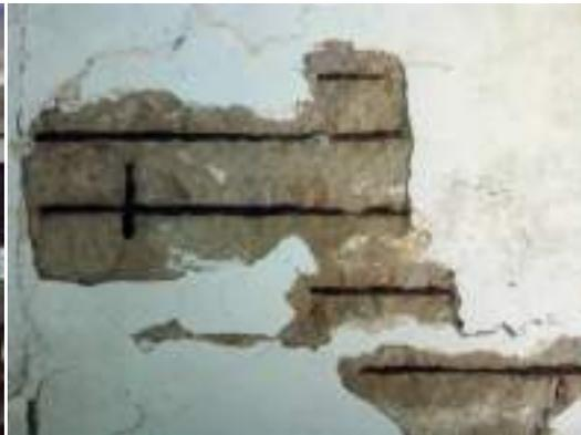
**Fig. 10: Exposed reinforcement in roof Slab**
