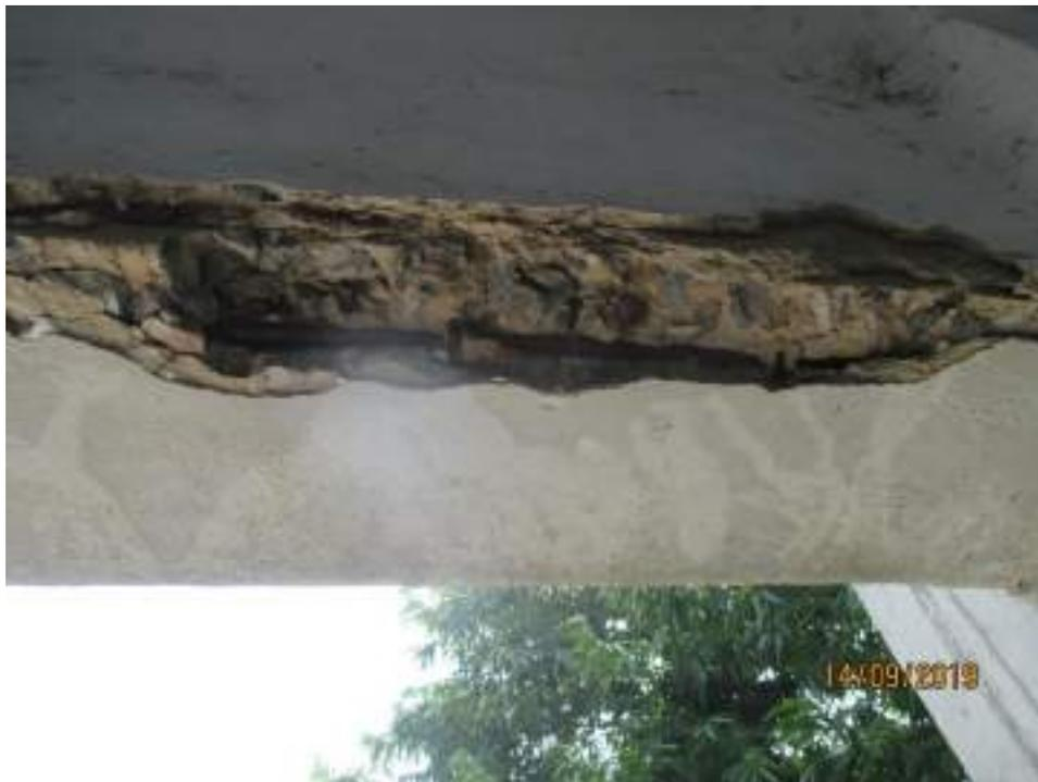
**Fig. 35 Larger size aggregates in RC Beams.**
