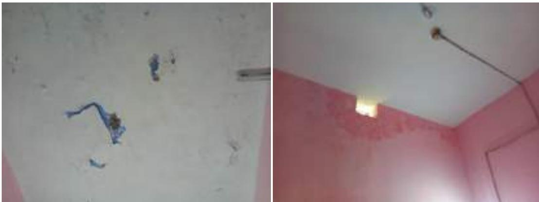
Fig. 21: Spalling of cover concrete and dampness in a renovated building of DS type.
