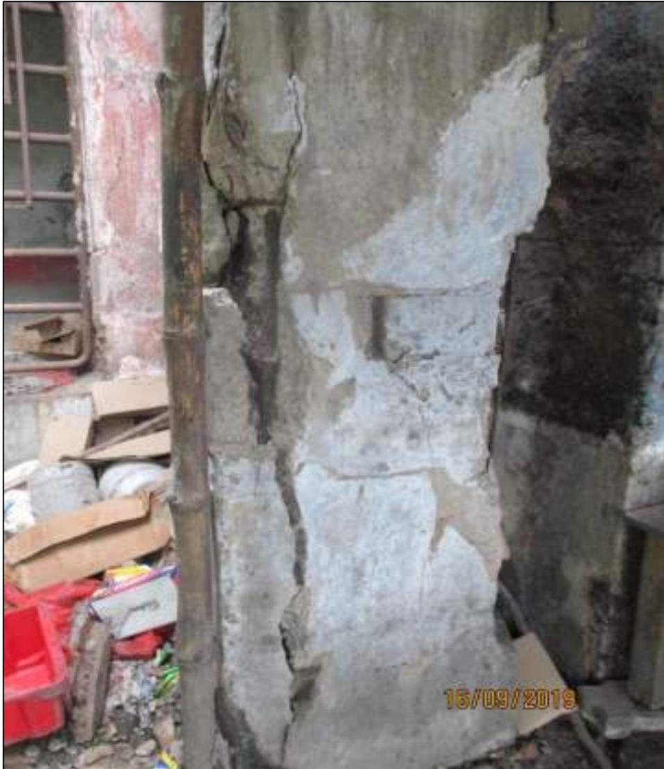
**Fig. 23 Spalling of cover portion from Column**
