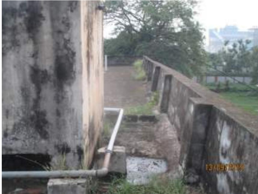
**Fig. 12 Inclined Parapet wall**
