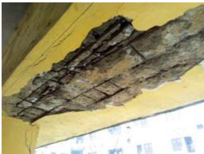
**Fig. 7: Exposed reinforcement in Cantilever slab of Officers Hostel 1 at Ground Storey**
