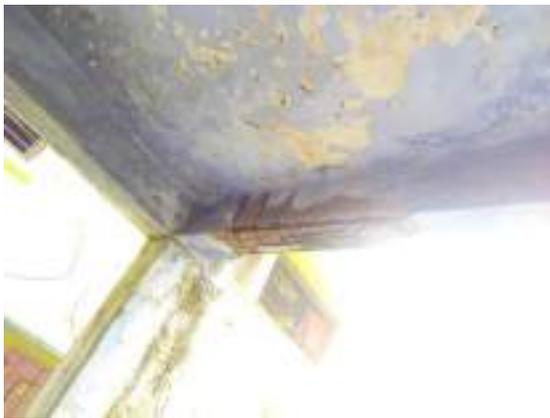
**(c) Portico beam corroded reinforcement**
