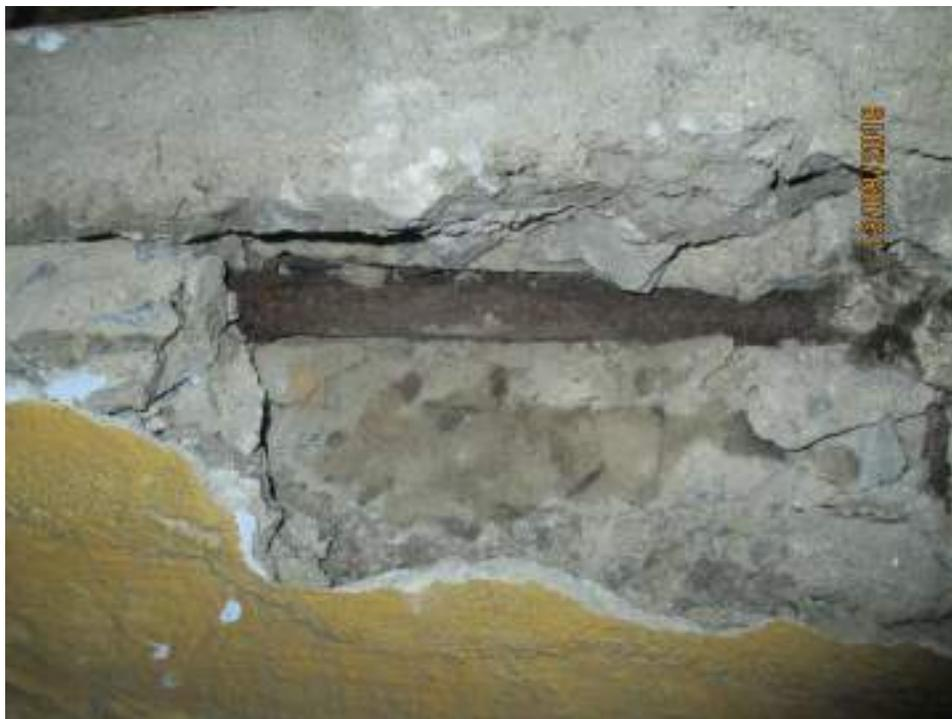
**Fig. 36. Fully crushed condition of core and main bars**
