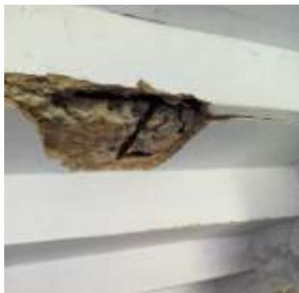
**Fig. 30: Corroded reinforcement in CISF building Stairs**
