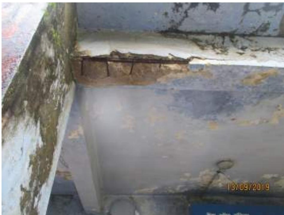
**Fig. 29 Spalling and Cracking of Core concrete**
