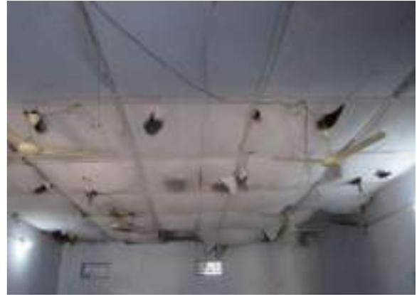
**Fig. 41: Damaged fall ceilings in class rooms**
