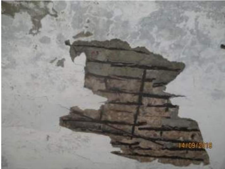
**Fig. 34 Severely Corroded and discontinued reinforcement in slab**
