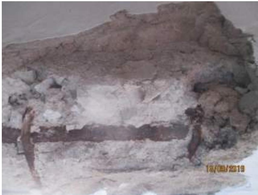
**Fig. 14 Collapsed stage of core concrete in beam**
