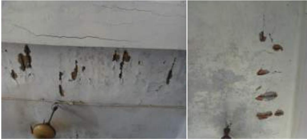
**Fig. 31: Exposed reinforcement in roof slab of CISF building**
