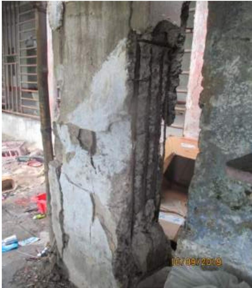
**Fig. 22. Damaged Column in the community center**
