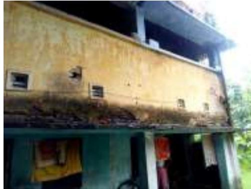
**Fig. 16: F Type Quarters (spalling/corrosion)**
