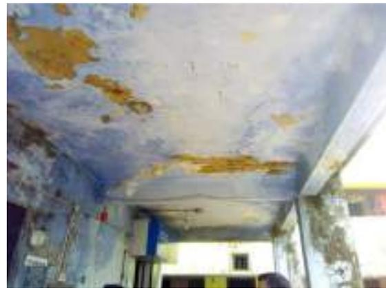
**(d) Portico slab corroded reinforcement**
