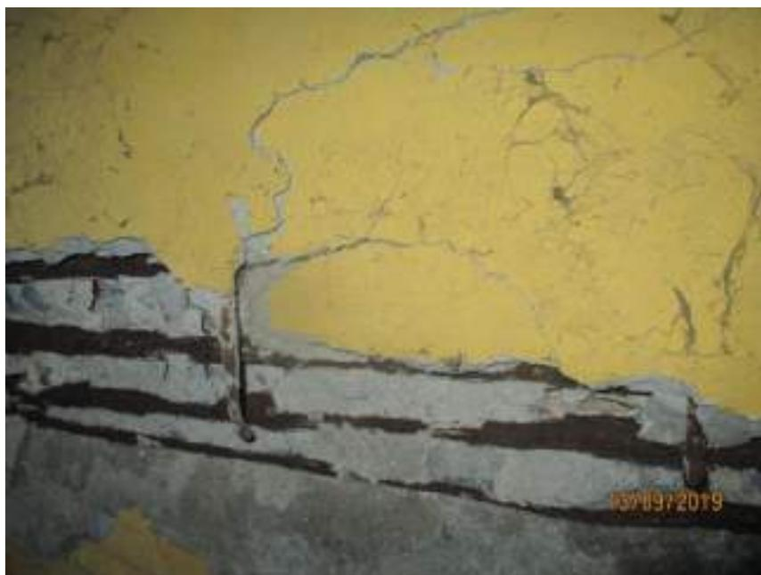
**Fig. 37 Damage due to corrosion in lintel and slab**
