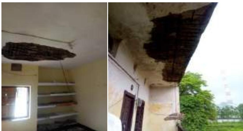
**Fig. 11: Exposed reinforcement and hanging reinforcement with a chunk of cover concrete**
