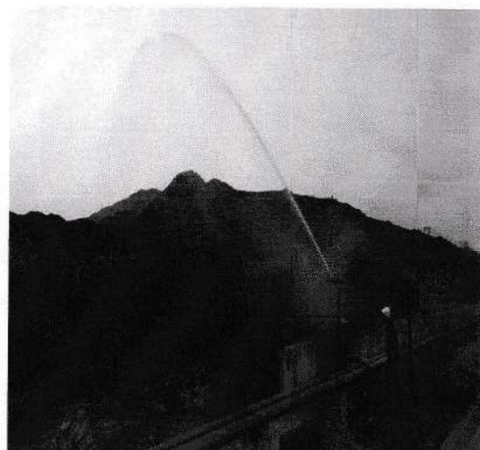
(Sprinkler at Coal Stack Yard)
