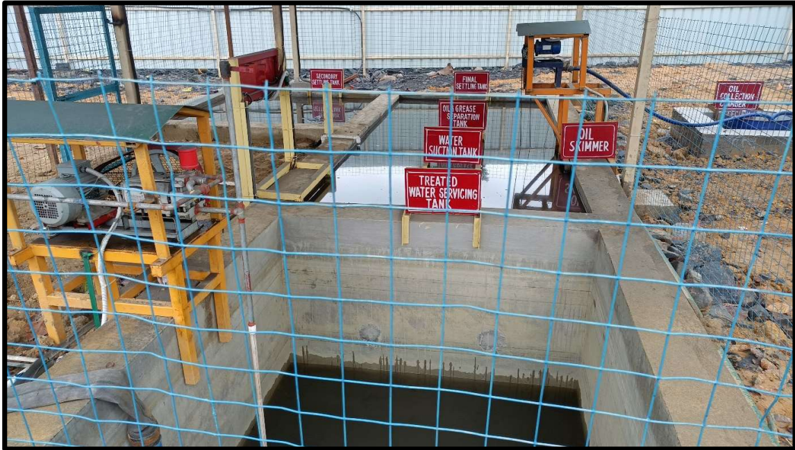
Picture : Oil & Grease Pit at Workshop
