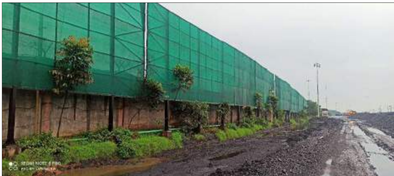
Photographs of Boundary wall with 20 ft. windscreen
