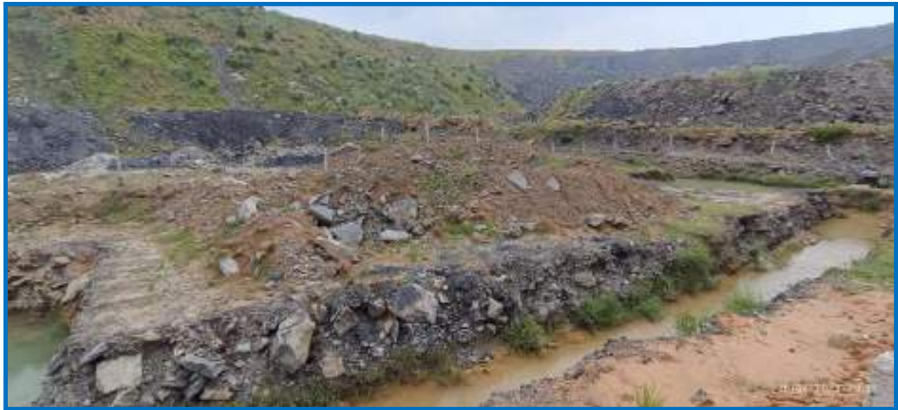
Photograph showing # Garland Drains and Siltation ponds along the OB Dump.
