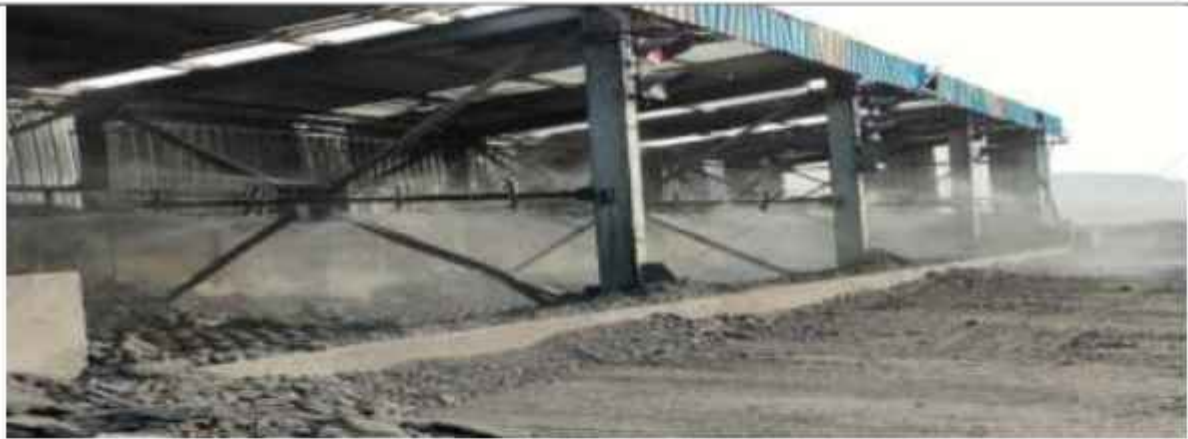
Dust Suppression at Receiving Hopper
