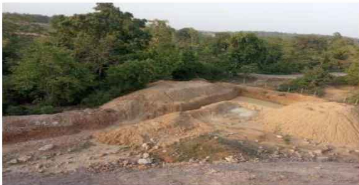
Garland Drain connected to settling pond
