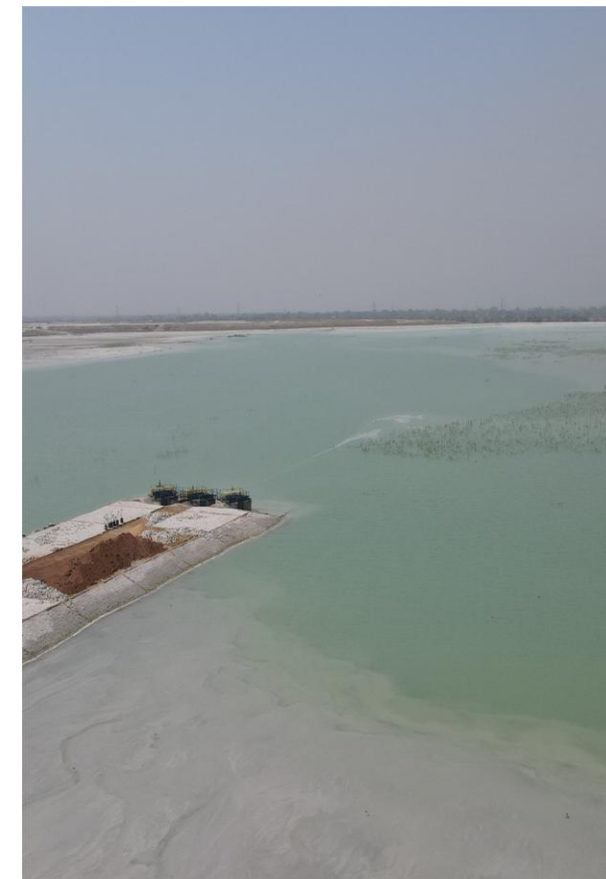
Ponding of charged Ash dyke
