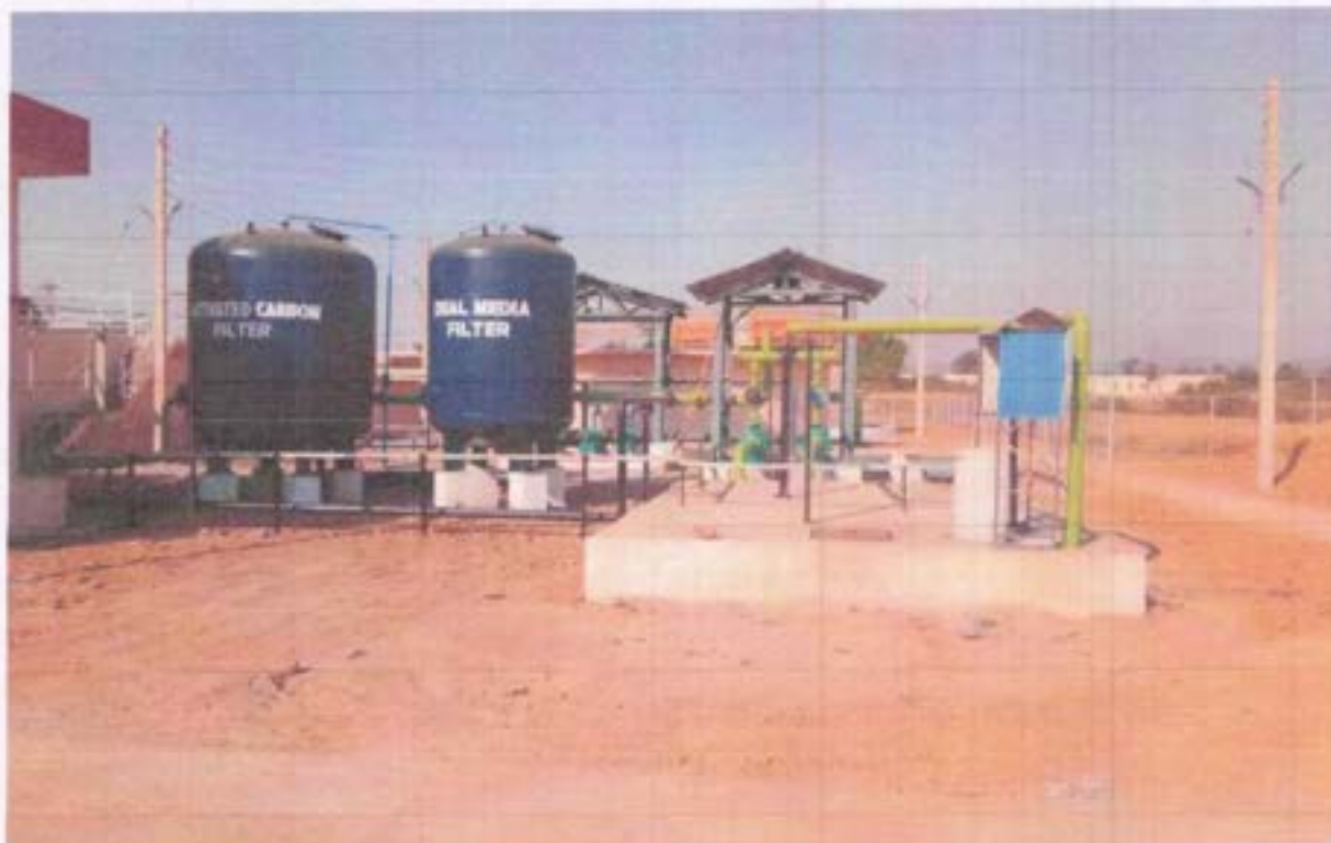
Photograph# 1.5 MLD STP for treatment of Sewage with the latest technology of MBBR System
