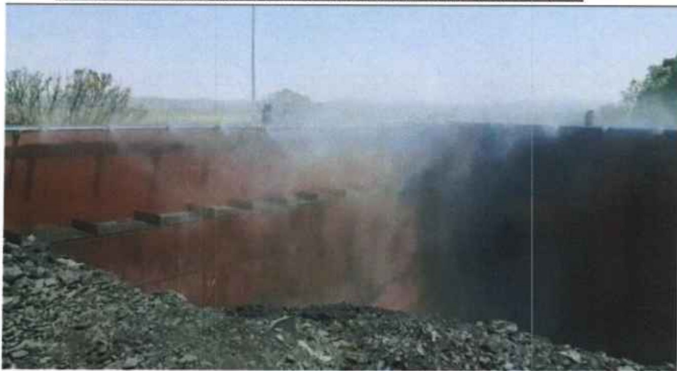
Water sprinkling system installed within the crusher unit
